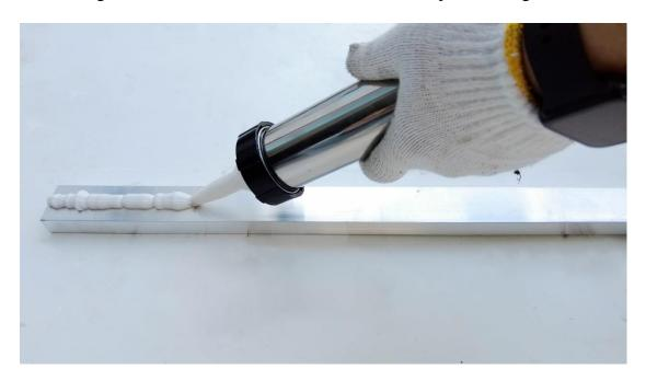
■ The two supports that are installed at the ends of each panel shall have a continuous bead of glue. The supports that are installed in the middle of the panel can be glue in sections. The bead length in these sections shall be minimum 200mm. The distance between supports and glue length in middle can be adjusted according to an assessment done of the site.
